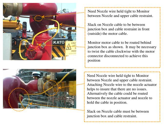
Note - Updated requirements no longer call for this mid-mounted junction box as of 2012. If desired, the cables are long enough to be connected directly to the bottom of the junction box, but holes will need to be punched and correct cable glands and hole plugs will be needed to be used to insure compliance with local requirements and codes.
