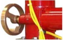
Hand wheels are provided for all three axis (horizontal, vertical, and nozzle) to operate the monitor in a power failure. See monitor manual for operating details.
